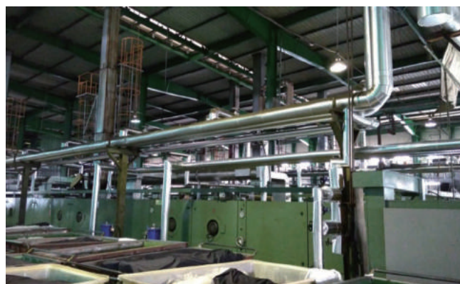
▲ Image 10 / Taiwan Cogen Corporation supplies medium-pressure steam to replace coal-fired thermal oil boilers in the dyeing and finishing industry
