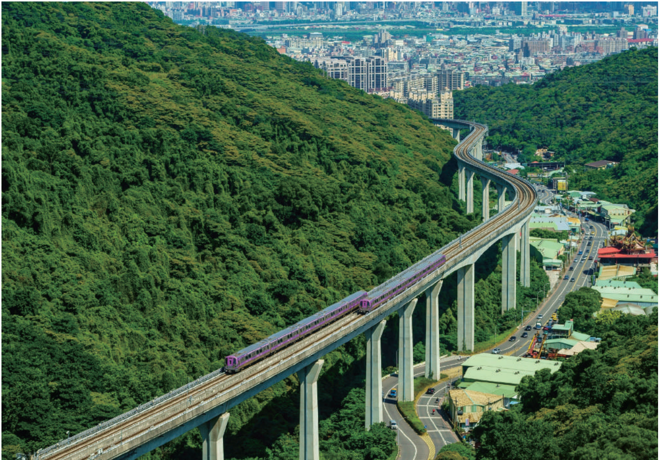
▲ Image 34 / High-pier viaduct in a water conservation zone
